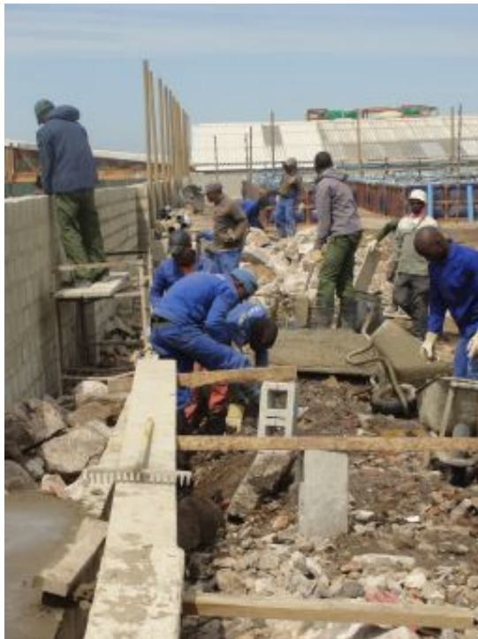
The retaining wall seen from the top of the platform
