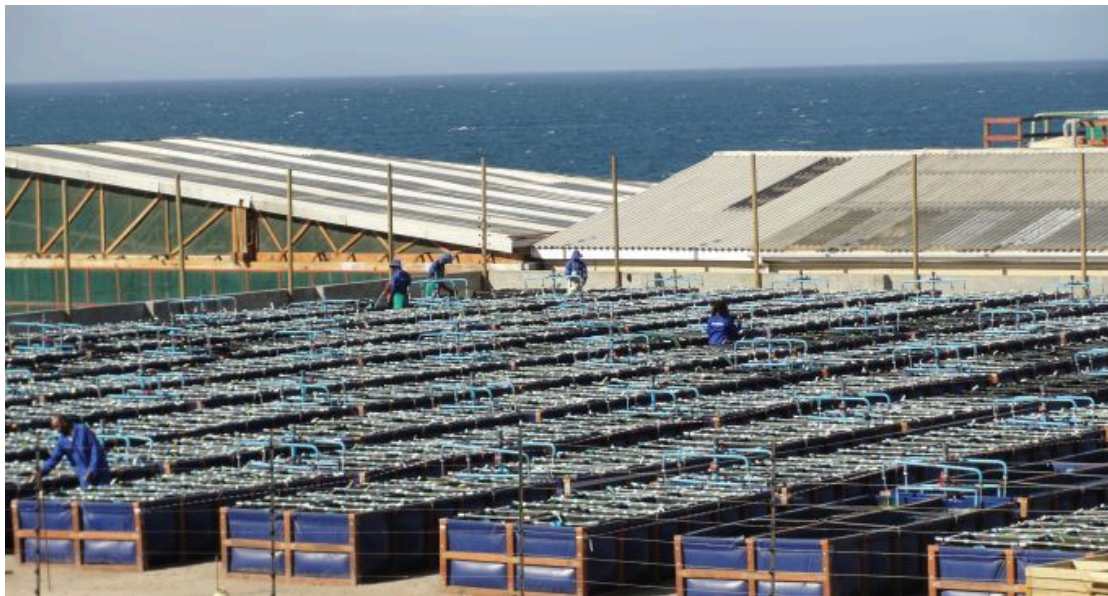
The completed section of Amaza 5
